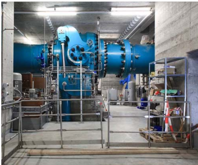
Figure 10. Main hydro-mechanical equipment Turbine Valve (l), Stator (r).
