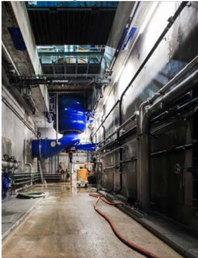
Figure 9. Main hydro-mechanical equipment. Pump (l), Pelton turbine (r).
